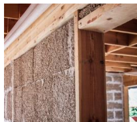
Figure 4. Detail for door opening.
