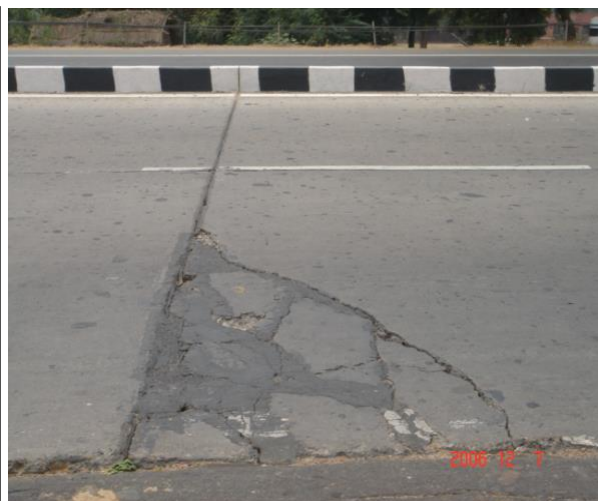
Photo 5. Corner Cracking
